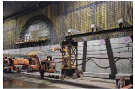
Installing support beams in the cavern for the new station beneath Grand Central Terminal. MTA
